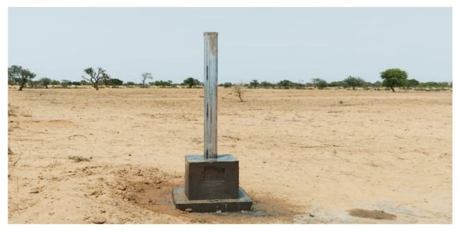
**Figure 3:** Picture of the Constructed Intermediate pillar along the Nigeria-Niger International Boundary
